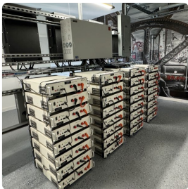
F. & B. Bracket hold up to 1*E-BOX 48100R, Stack up to 4*E-BOX 48100R
