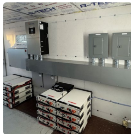
R-Bracket hold up to 8*E-BOX 48100R
